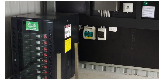
Rack-mounted lithium battery
